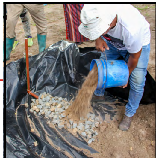
Professor Luderlândio Andrade, from UFCG, demonstrates how to set up the economic construction site in Misungwi district in November 2022. Photo: WFP
