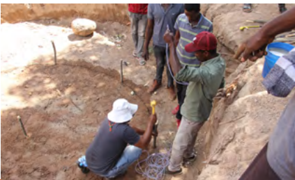
Figure 10: Demarcating the bottom of the cistern to build the floor
