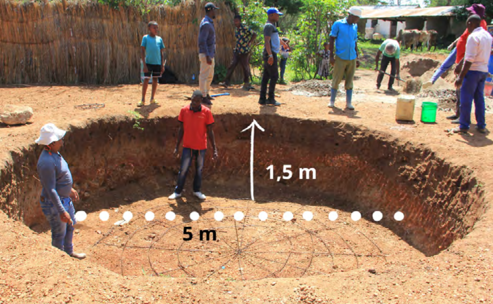
Figure 2 – Excavation Dimensions
