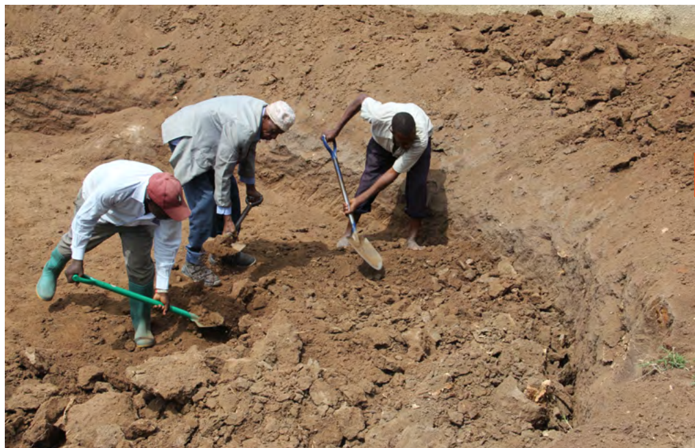
Figure 3 – Excavation of the Foundation
