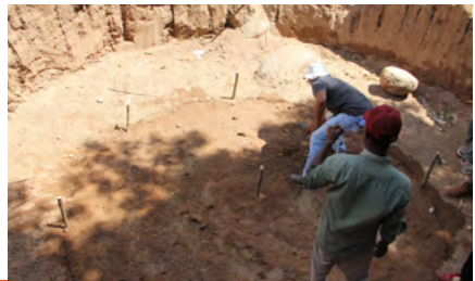
Figure 10: Demarcating the bottom of the cistern to build the floor
