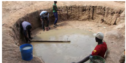
Figure 11: Level marking and floor construction
