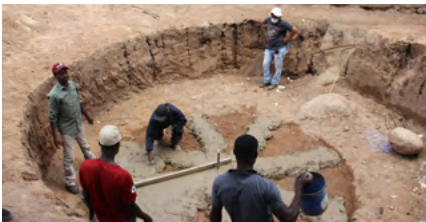
Figure 11: Level marking and floor construction
