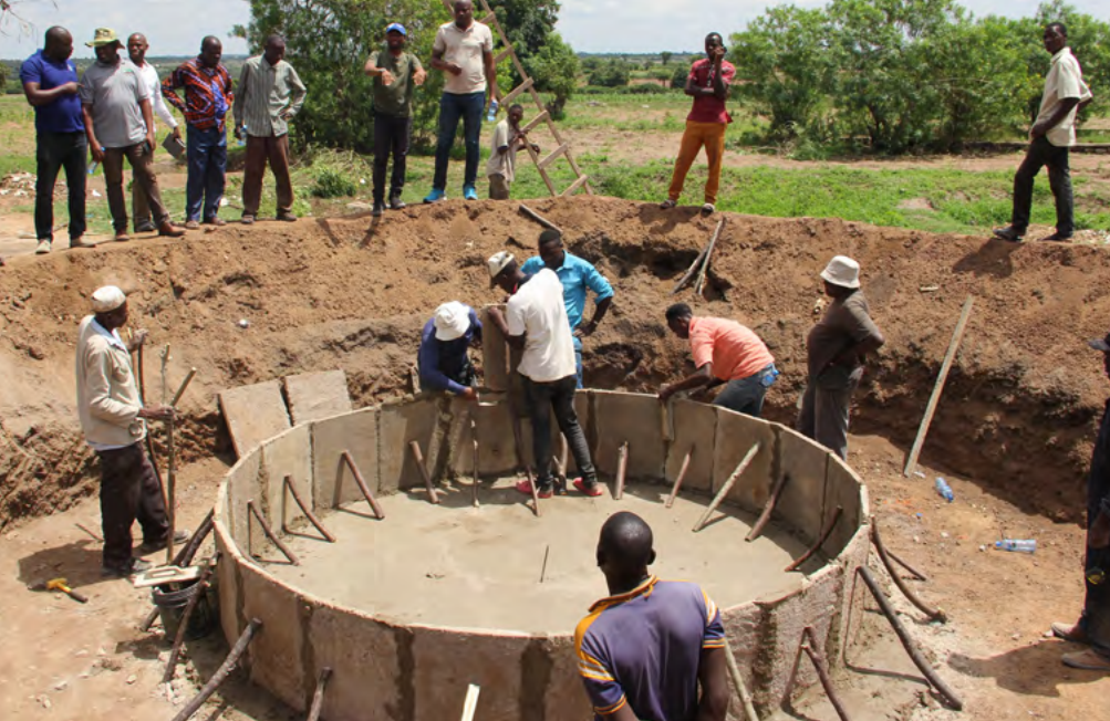
Figure 14 – Assembly of the 1st. Row of Plates
