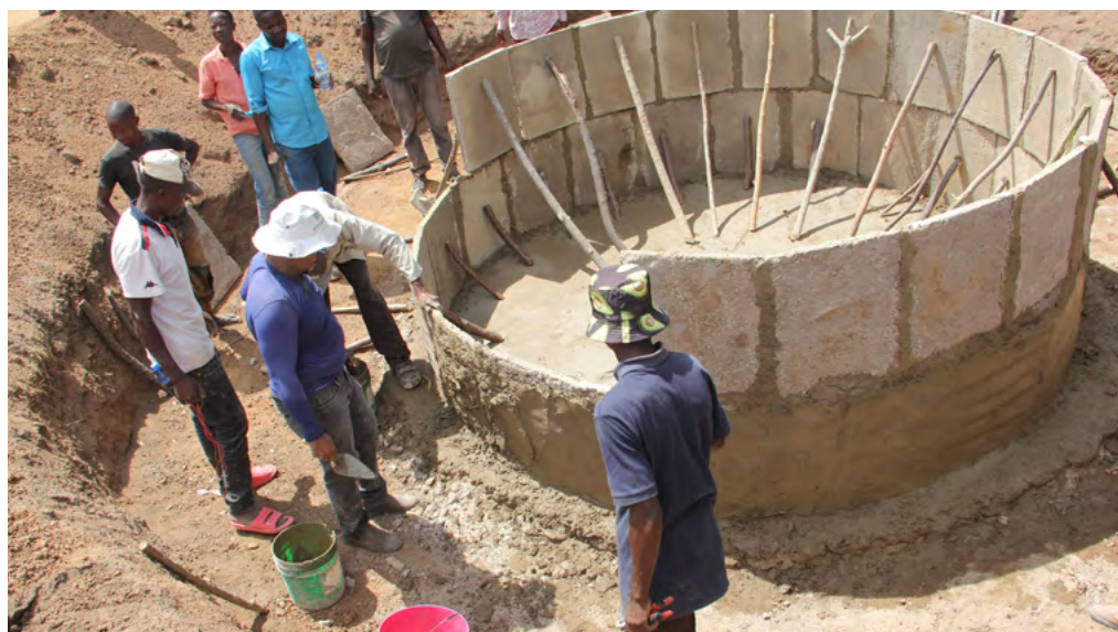
Figure 15 – Details of the Assembly of the 2nd. Row
