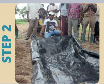
With a canvas of 100 to 200 microns, line the patch taking care with the levelling so that there are no holes or mud puddles. If you are going to step on the tarp, be careful not to tear it. You can bend the sides of the canvas, cut the leftovers carefully, or place stones on the sides, in order to have a better patch.
