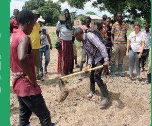
Dig a hole 1 metre wide and 20 centimetres deep. The length may vary as needed. After the excavation do the levelling of the soil.
